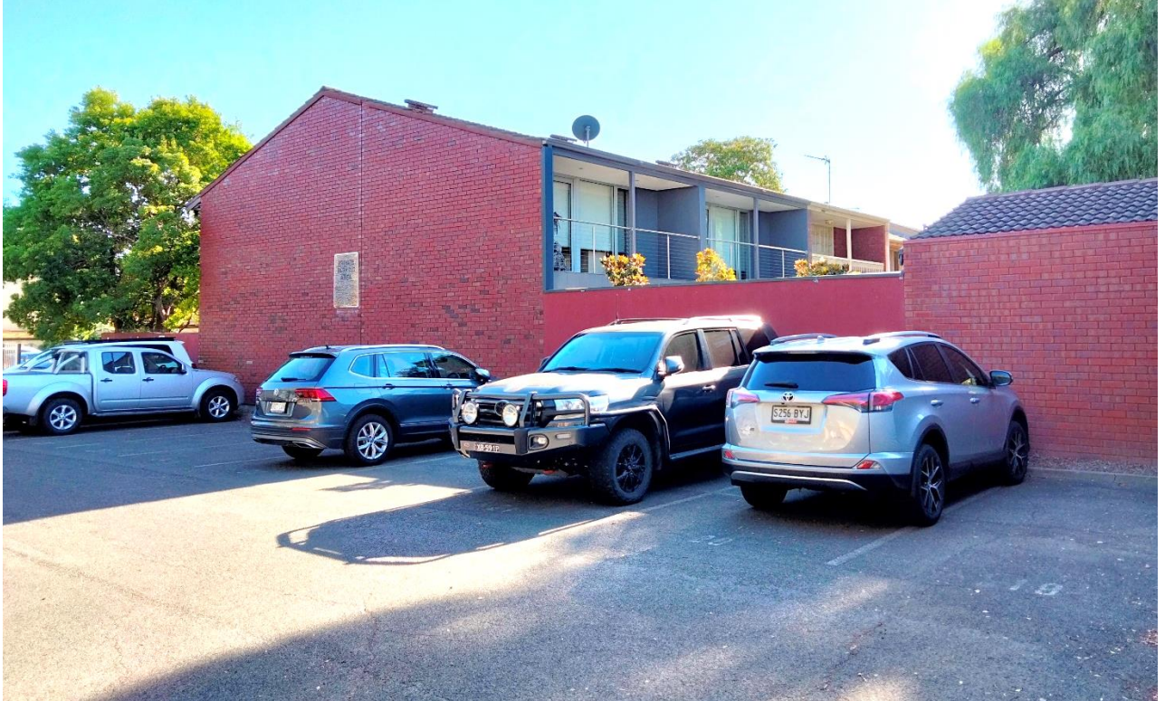
Photo 3.4 – Adjoining residential dwellings to the east
